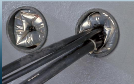
Inflatable wrap-around duct seals
